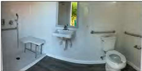
Panorama of finished modular shower/bathroom.
