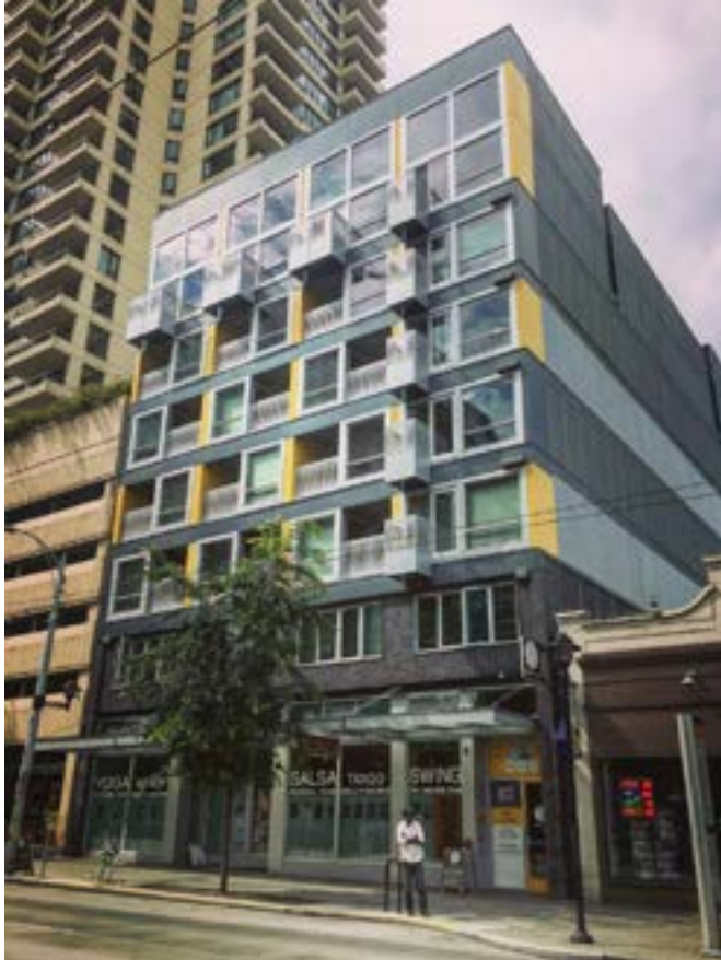
OneBuild's 'N' Habitat seven-story mixed-use development
